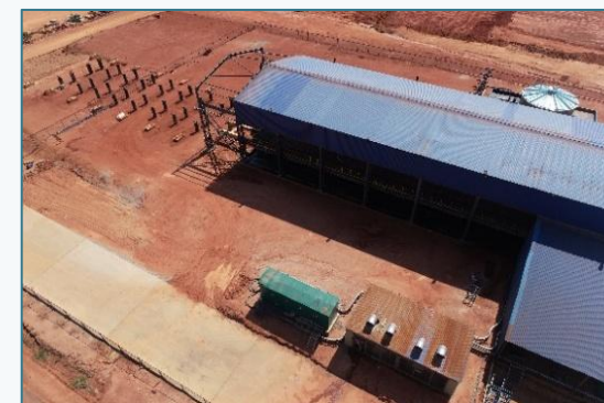
Electrowinning plant extension
