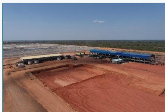
SX/EW plant & expansion groundworks
